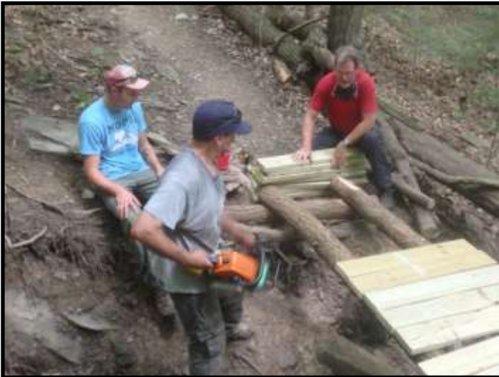
Dave Pigeon, with chainsaw, Don Orr, right, and Matt Forshey lay bridge planking. Photo by Mal Provost
