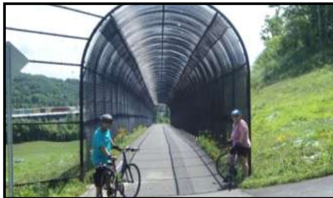
Jan and Marc Limeri prepare to enter the tunnel on the recently completed section of the Zim Smith bike trail in Saratoga County. Photo by Roy Keats
