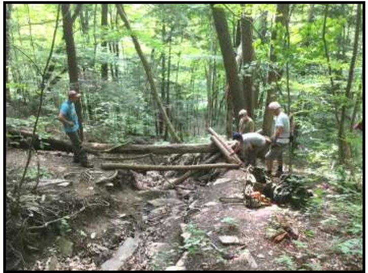
The beginnings of the bridge. Photo by Kathy Fisher
